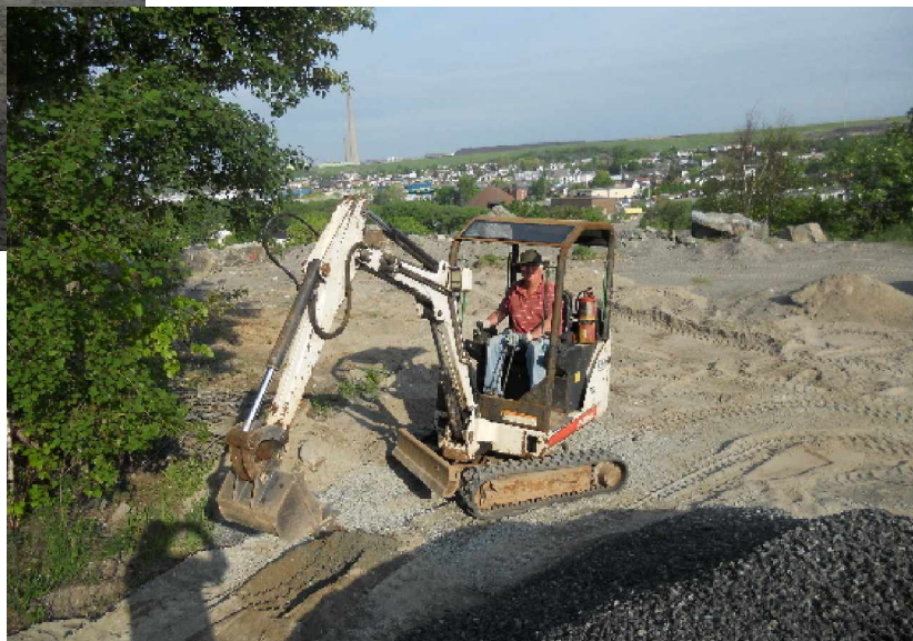
Bro. Roger Kitching preparing a drainage trench
